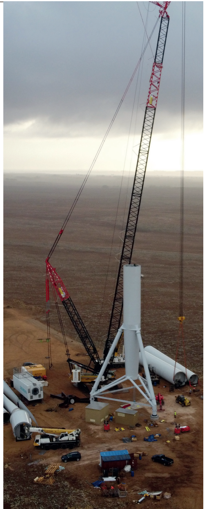
A world premiere by InnoVent: Three individual footings instead of a concrete swimming pool, reducing the greenhouse gas emissions by 7 to 10
